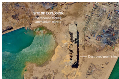
Mapping Damage in Beirut
